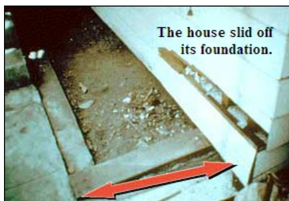
Slika 19: Zdrs konstrukcije med potresom ( http://geot.civil.metro-u.ac.jp/archives/eq/ ) Fig. 19: Sliding movement of a house atop the foundation during an earthquake ( http://geot.civil.metro-u.ac.jp/archives/eq/ )
