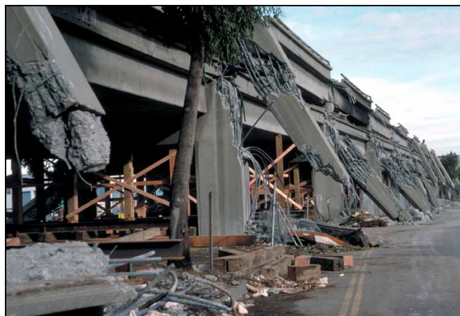
Slika 1: Posledice potresa ( http://geot.civil.metro-u.ac.jp/archives/eq/ , 20.06.2007) Fig. 1: Aftermath of an earthquake ( http://geot.civil.metro-u.ac.jp/archives/eq/ , 20.06.2007)
