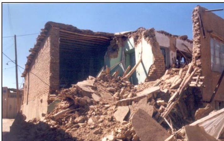
Slika 4: Posledice potresa ( http://geot.civil.metro-u.ac.jp/archives/eq/ , 20.06.2007) Fig. 4: Aftermath of an earthquake ( http://geot.civil.metro-u.ac.jp/archives/eq/ , 20.06.2007)
