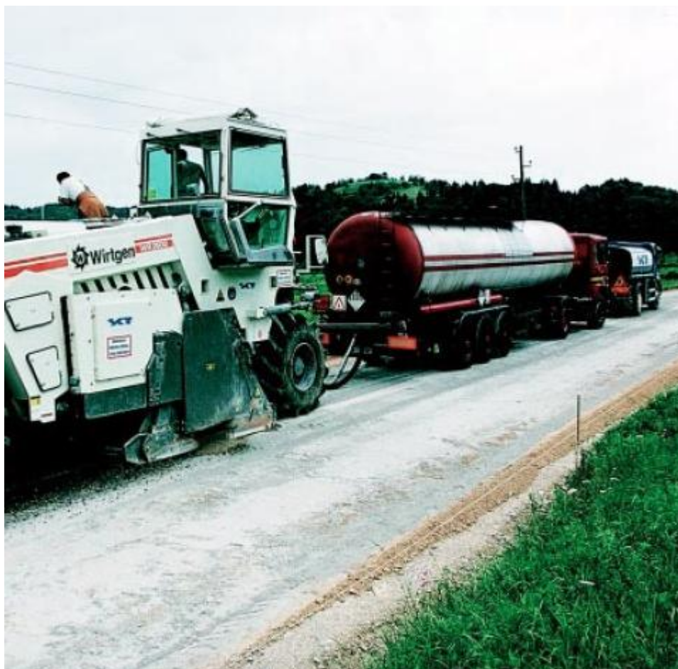
Slika 23: Reciklator, cisterna z bitumnom, cisterna z vodo [37]
