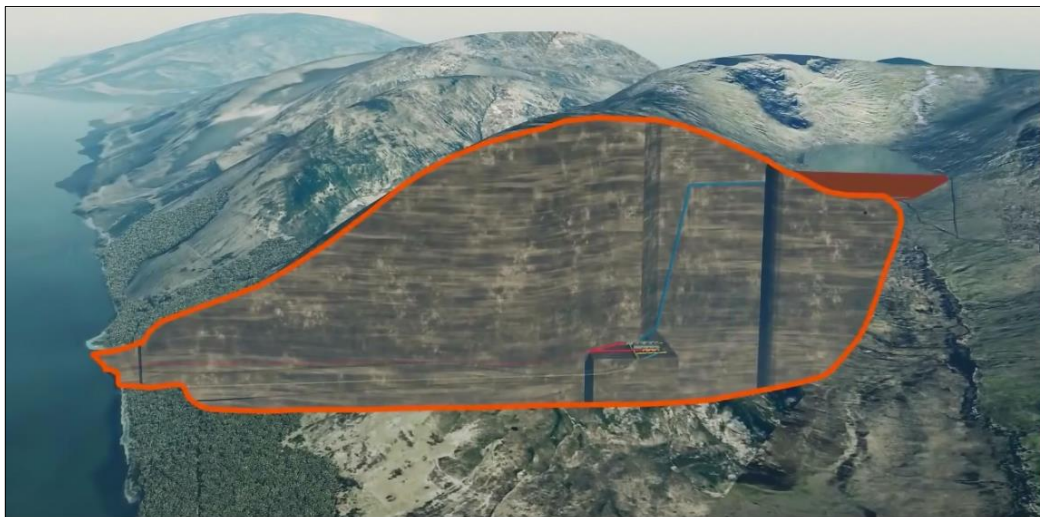
Slika 44: Prečni prerez ČHE Coire Glas (vir: Coire Glas..., 2015) Figure 44: Section of PSH Coire Glas (source: Coire Glas..., 2015)
