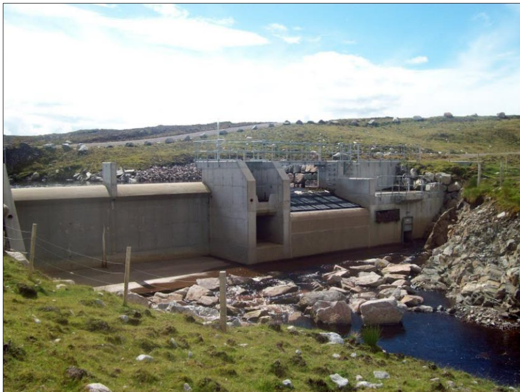
Slika 59: Nov vtočni objekt HE Glendoe (vir: Walkinghighlands, 2015) Figure 59: New intake on the Glendoe aqueduct (source: Walkinghighlands, 2015)
