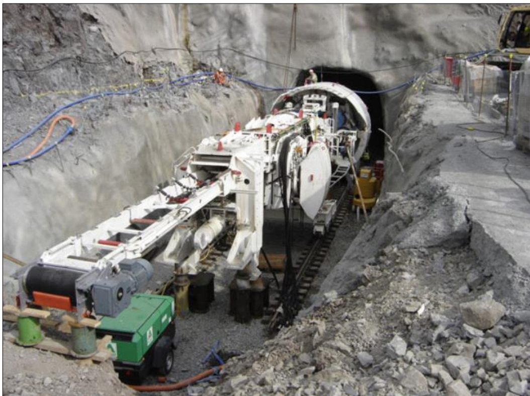
Slika 54: Tunelni vrtilni stroj Eliza Jane 2 (vir: Glendoe: in the..., 2015) Figure 54: Tunnel boring machine (TBM) Eliza Jane 2 (source: Glendoe: in the..., 2015)
