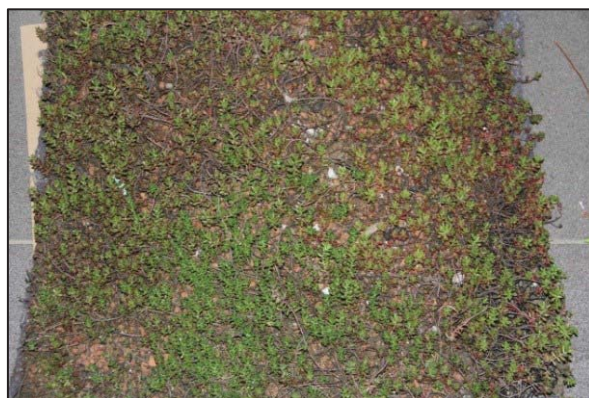
Slika 5: Vegetacijska preproga Sedum-moss na strehi 1 (Vir: avtor) Figure 5: Vegetation carpet Sedum-moss of the roof 1 (Source: author)
