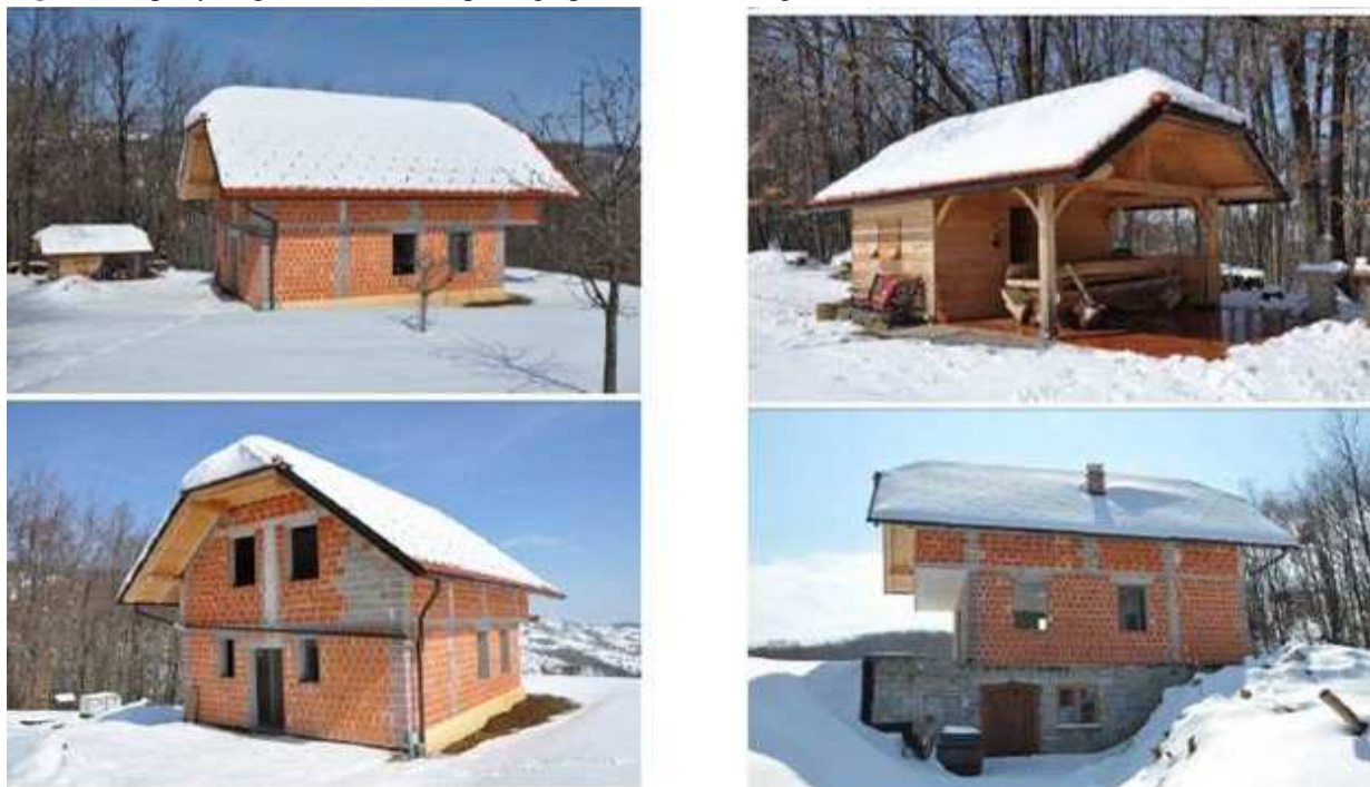
Fig. 33: Property Register–distinctive photographs of the building
