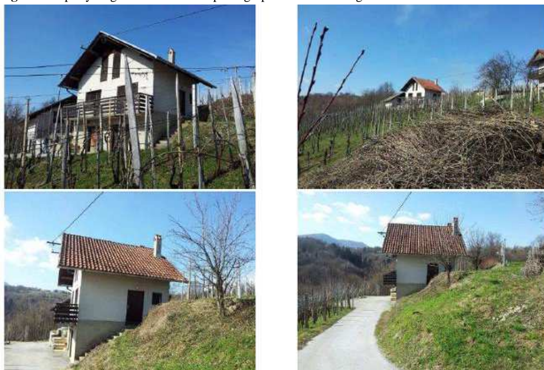
Fig. 43: Property Register – distinctive photographs of the building
