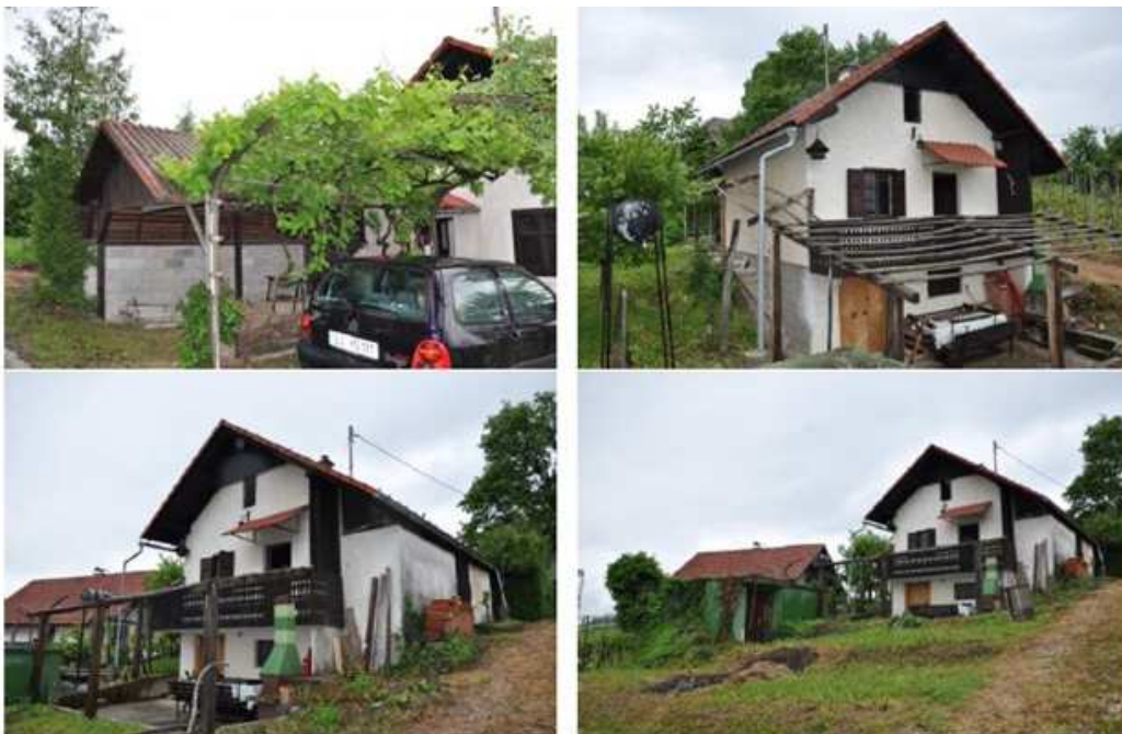
Fig. 37: Property Register – distinctive photographs of the building
