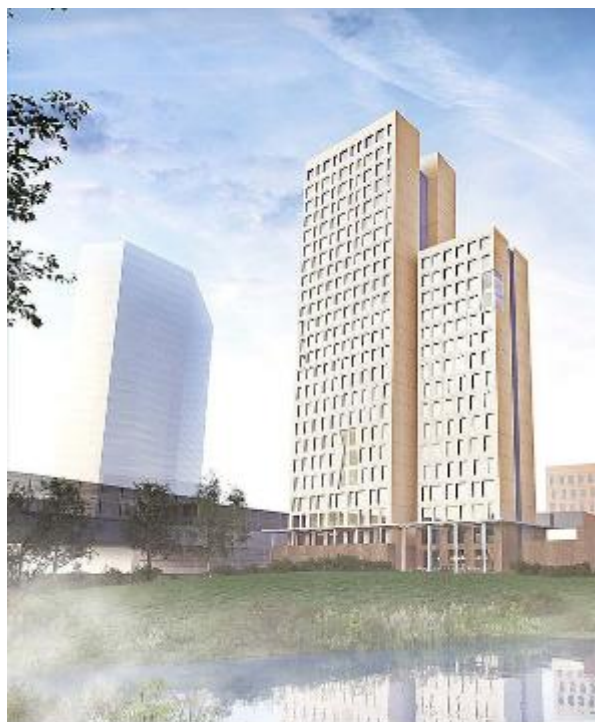
Slika 23: Stolpnica Hoho Tower (Timber design and technology)
