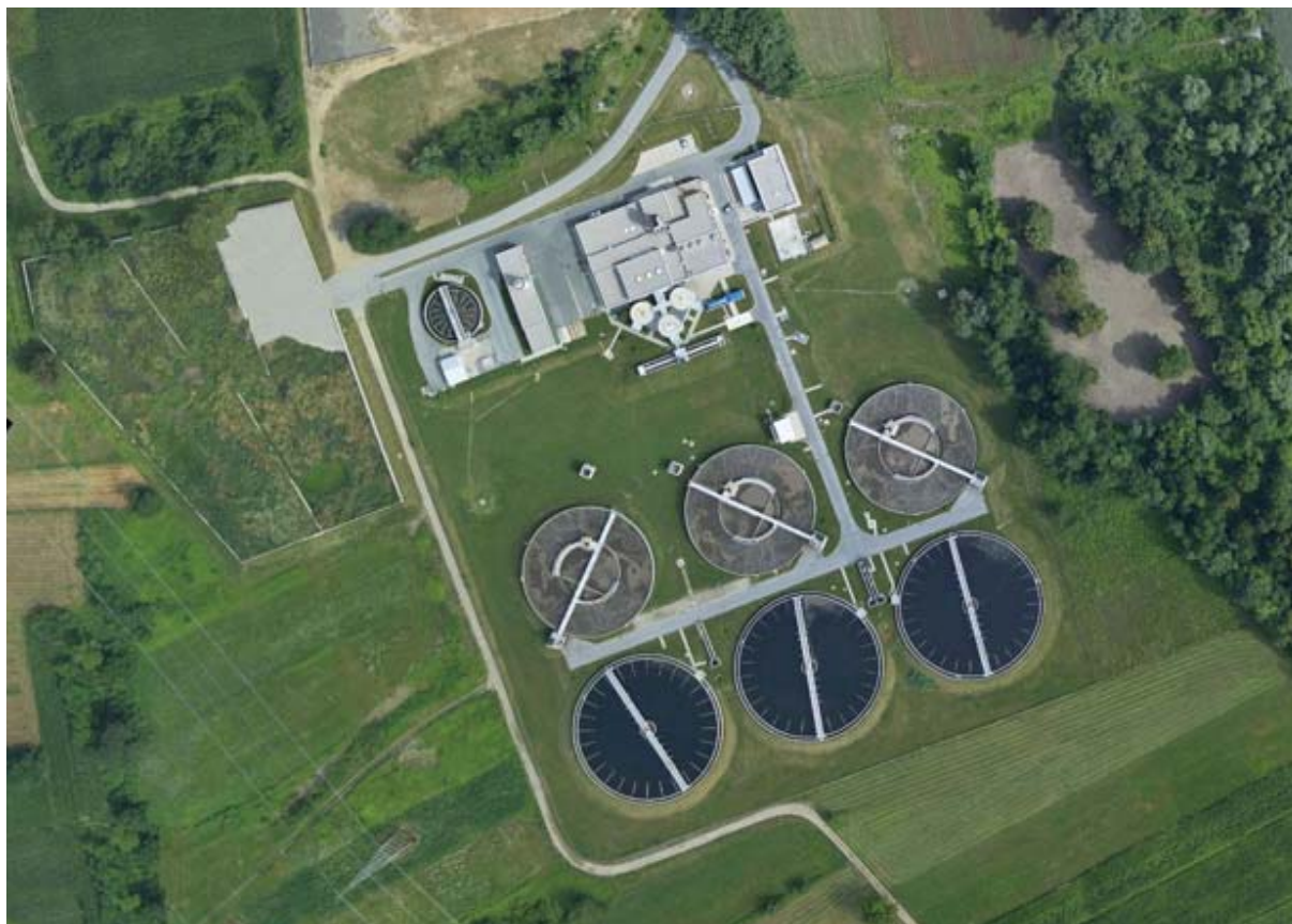
Slika 3: Centralna čistilna naprava Maribor (Aquasystems, 2016) Figure 3: Central wastewater treatment plant in Maribor (Aquasystems, 2016)
