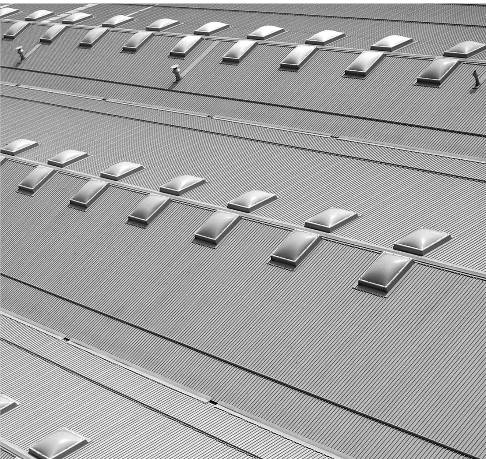
Ognjevarni STREŠNI paneli Trimoterm SNV
