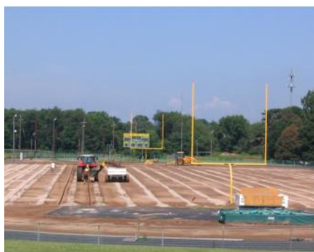
Slika 25: Namestitev cevne drenažnega sistema (Sports Turf Managers Association, 2016, part three)
