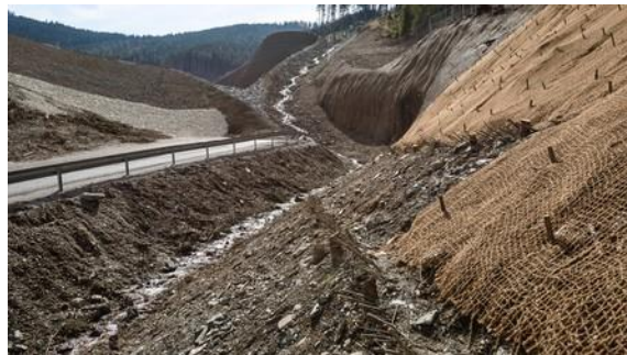
Slika 36: Korito prestavljenega potoka dolvodno glede na deponijski prostor Figure 36: The bed of the displaced brook downstream in relation to the landfill space (vir: Bildergalerie Baustraßen Gemeinde Spital & Vorarbeiten Deponie Longsgraben http://www.oebb.at/infrastruktur/ , 2014)
