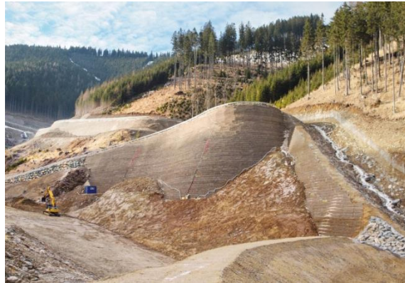
Slika 34: Pogled na armirano brežino iz smeri vznožja deponijskega prostora Figure 34: View of the reinforced slope from the direction of the foot of landfill space (vir: Schmidt, S., 2014. Geosynthetics 32, 3: 14-18)
