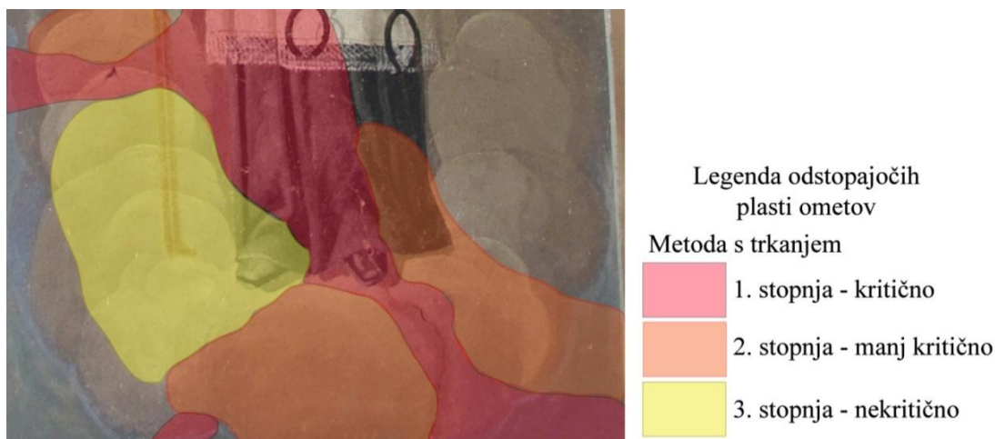
Slika 5.3: Označeni del odstopajočih plasti ometov z metodo s trkanjem. Figure 5.3: Marked detached plaster layers evaluated by the tapping method.
