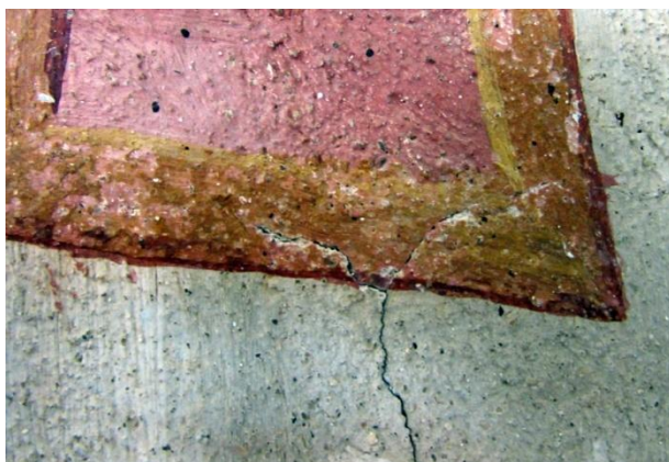
Slika L.4: Razpoke na stenski sliki. Figure L.4: Cracks in the mural painting.
