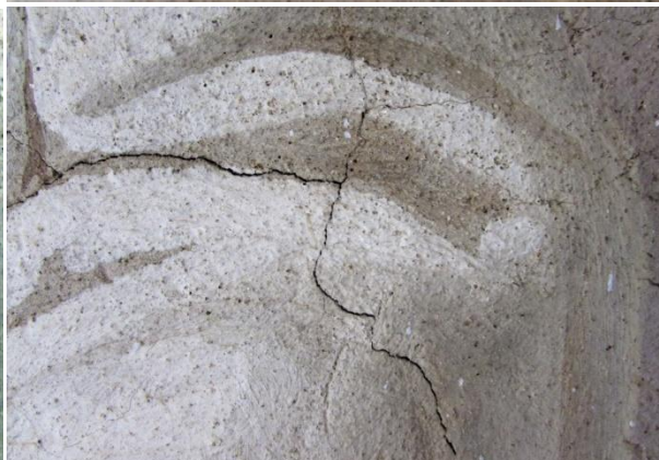
Slika L.4: Razpoke na stenski sliki. Figure L.4: Cracks in the mural painting.
