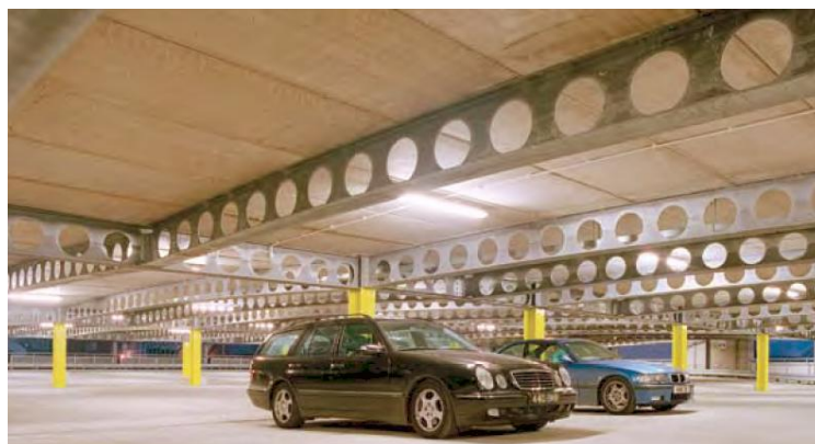
Slika 18.3: Uporaba satastih nosilcev v Capitol Car Park, Douglas, Isle of Man (Cellular Beam Design Guide, 2008)
