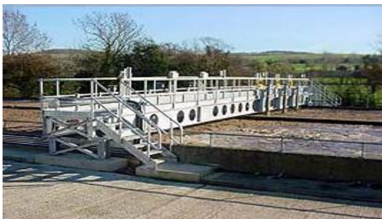
Slika 18.7: Ivinghoe Scraper Bridge (Cellular Beam Design Guide, 2008)
