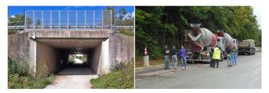
Figure 6: The instrumented underpass (left), and the static weighing of vehicles (right).
