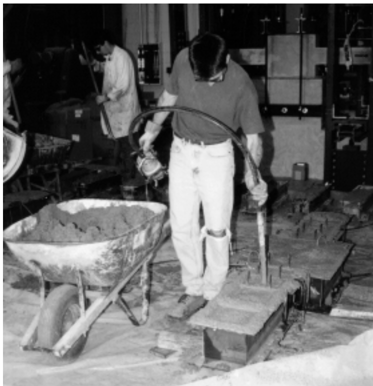
Figure A.24. Concrete being vibrated inside the metal forms.
