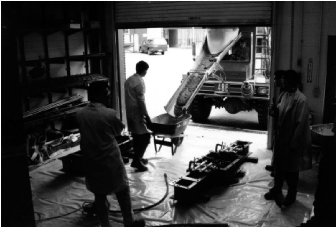
Figure A.23. Concrete being delivered by mixer truck.
