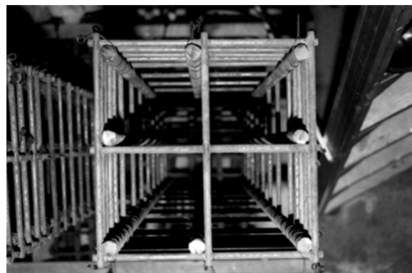
Fig. 2(a)—8-bar reinforcement arrangement with 4-cell grids.
