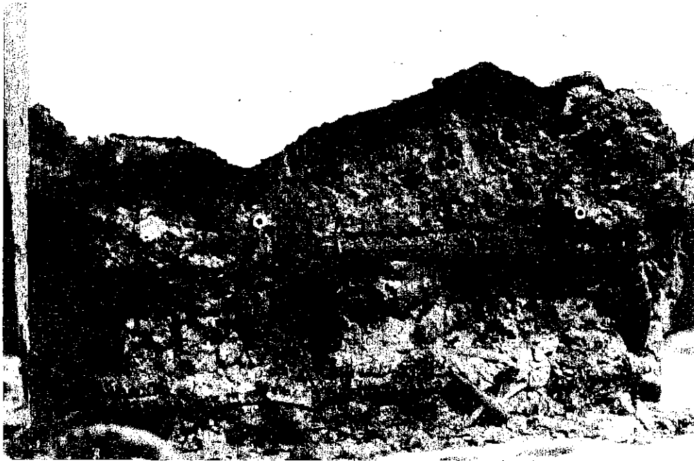
(b) The 'U' bar interior cross ties are still effective.
