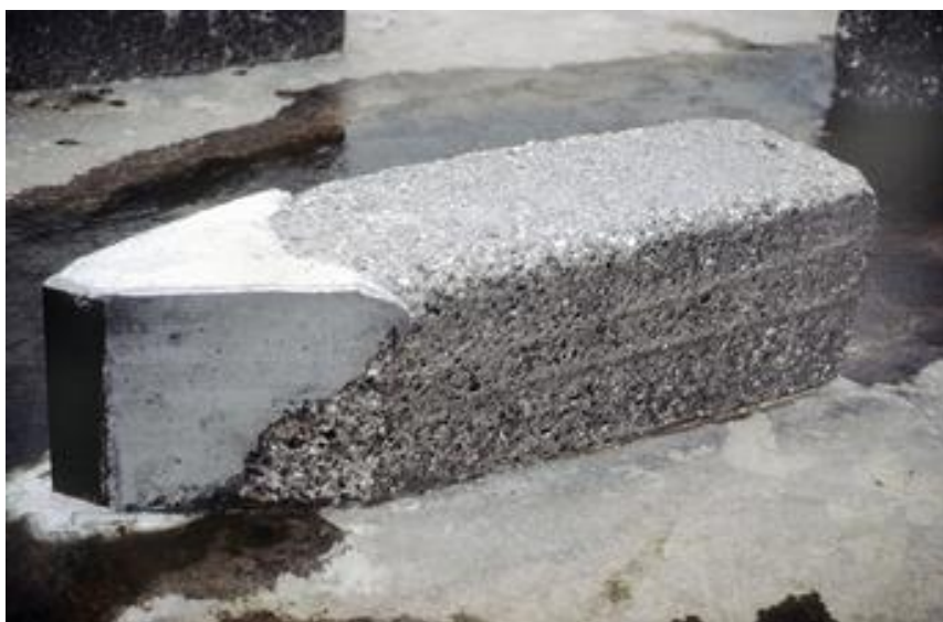
Slika 11: Poškodovan razbijač (International Water Power & Dam Construction)
