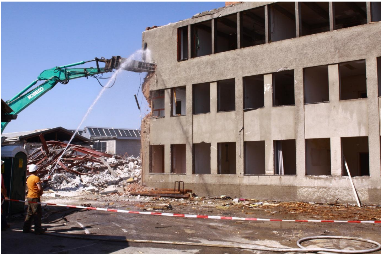
Figure 3. Demolition works of the existing building (NFL, 2010)
