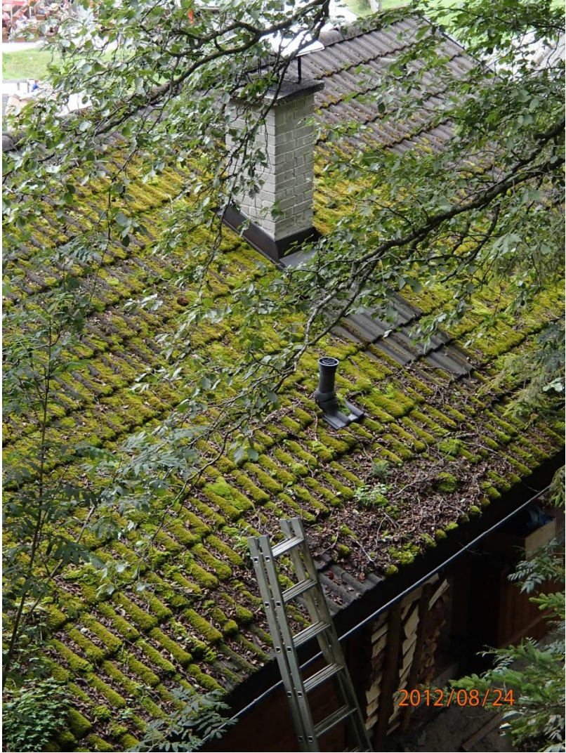
Fig. No. 1: Sloping roof before maintenance
