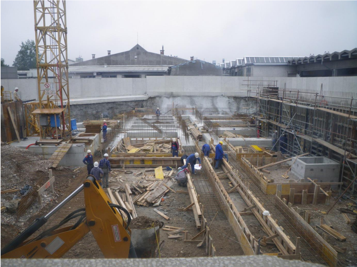
Figure 5. Implementation of foundations (NFL, 2010)
