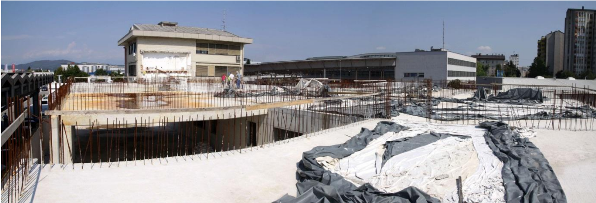
Figure 6. Panoramic view of the completed ground floor slab (NFL, 2010)
