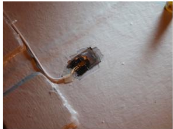
Figure 9: Viaduct Lešnica – one of the measuring points on the lower part of the construction
