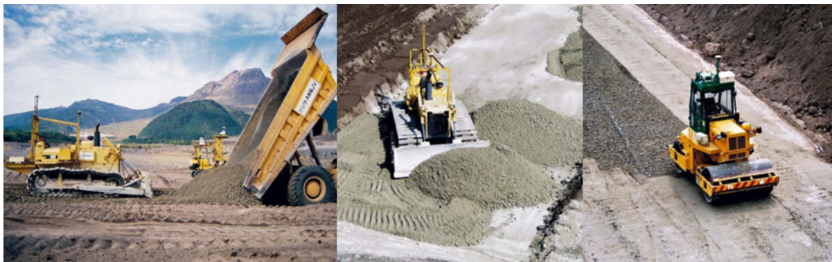
Slika 13: Proces vgradnje RCC valjanega betona (Unzen Restoration Project Office, 2007)
