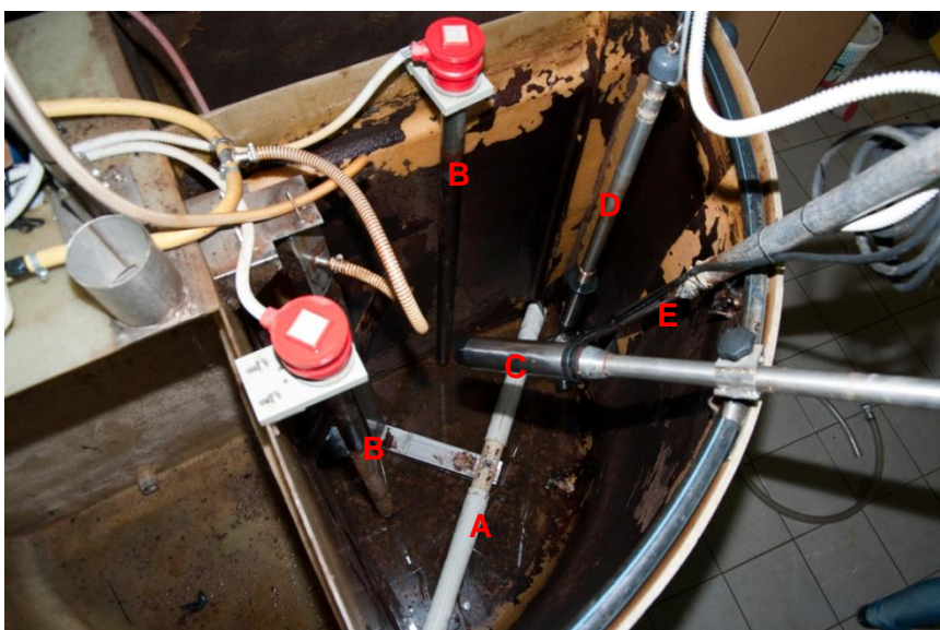
Slika 13: Biološki del pilotne čistilne naprave Picture 13: The biological part of the pilot plant
