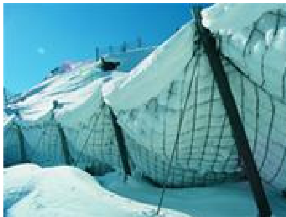
Fig. 2 Filets paravalanches surchargés Fig. 2 Overloaded avalanche protection nets
