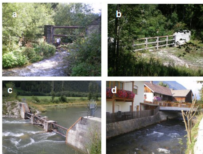
Fig. 9 Wood retention check-dams and several bridges are present in most of the Rienz tributaries.
