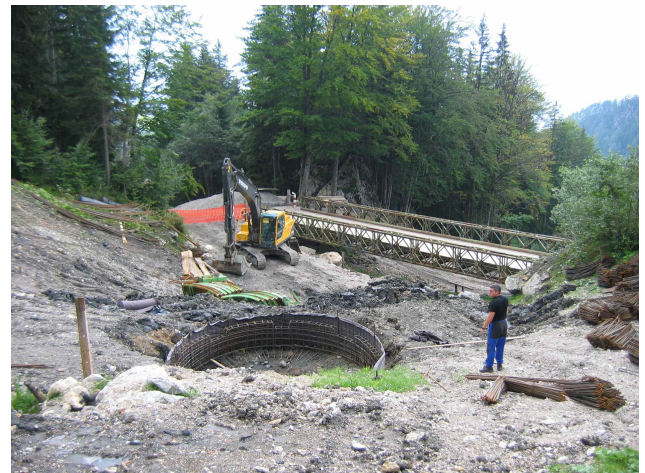
Fig. 16. Execution of a RC well just above the pontoon bridge.
