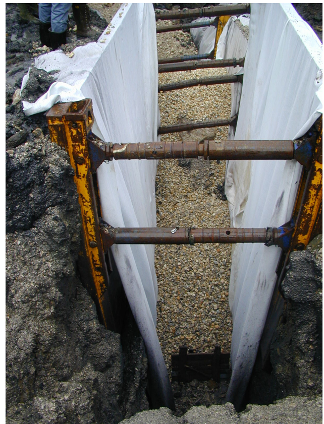
Fig. 13. Detail of deep drain trenches.
