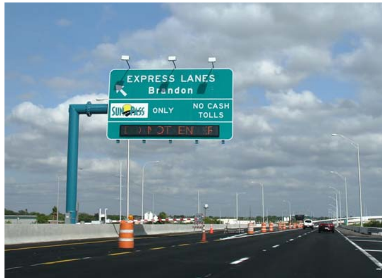
Slika 2-4: Primer ITS ukrepa spremenljive oblike infrastrukture, Tampa Bay Reversible Express Way (THEA, 2011)
