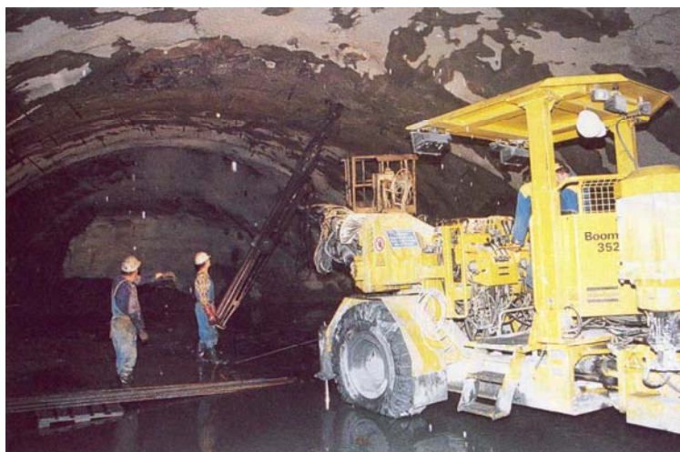
Slika 15: Vgradnja IBO sider (Vir: Teh. Informator SCT: December 1999)
