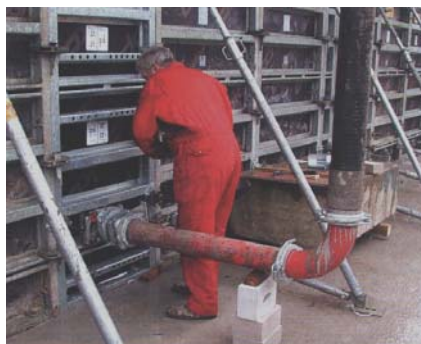
Slika 2.2: Vgrajevanje SCC s črpanjem ob dnu opaža Fig. 2.2: Casting of SCC by pumping from below
