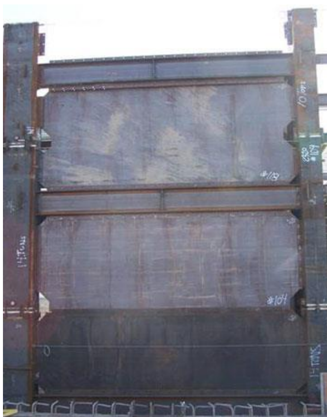
Slika 5: Primer strižne stene ( http://www.nyase.com/lalive.php )
