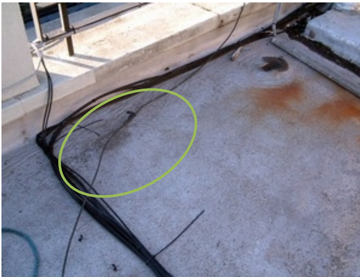
Slika 28: Primer lezenja (when flat roofs fail, 2016).
