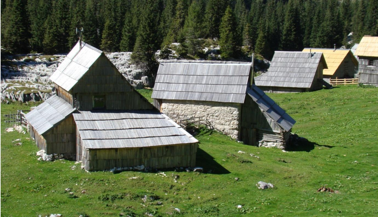
Slika 20: Uporaba lesene kritine na zidanih in lesenih stanovih na pl. Laz Figure 20: Shingle covered roofs on brick-built and wooden herdsman's cottages on the Laz Plateau
