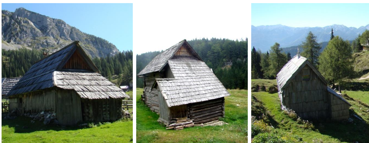
Slike 16, 17 in 18: Dodajanje prostorov ob osnovni objekt na planinah Laz (levo), Blato (v sredini) in Krstenica (desno) Figures 16, 17 and 18: Adding extra rooms to the main building on the plateaus Laz (left), Blato (middle) and Krstenica (right)
