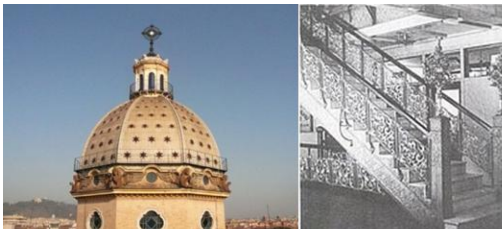
Slika 18: Aluminijasta kupola cerkve San Gioacchino in aluminijaste stopnice v Monadnocku ( http://www.twrbifolds.co.uk/timeline-aluminium-building-construction-1800s/ )
