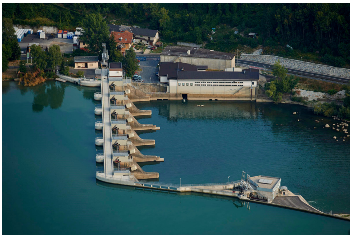
Slika 14: Jez Melje in mala HE Melje (Zaključena prenova HE Zlatoličje, jezcu Melje in izgradnje MHE Melje URL, 2014) Figure 14: Dam Melje and small hydroelectric power plant Melje (Zaključena prenova HE Zlatoličje, jezcu Melje in izgradnje MHE Melje URL, 2014)
