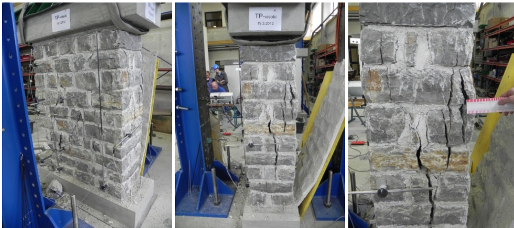
Figure 3.22: Damage of the wall with through stones after test TP-visoki Slika 3.22: Poškodbe na povezanem zidu po testu TP-visoki
