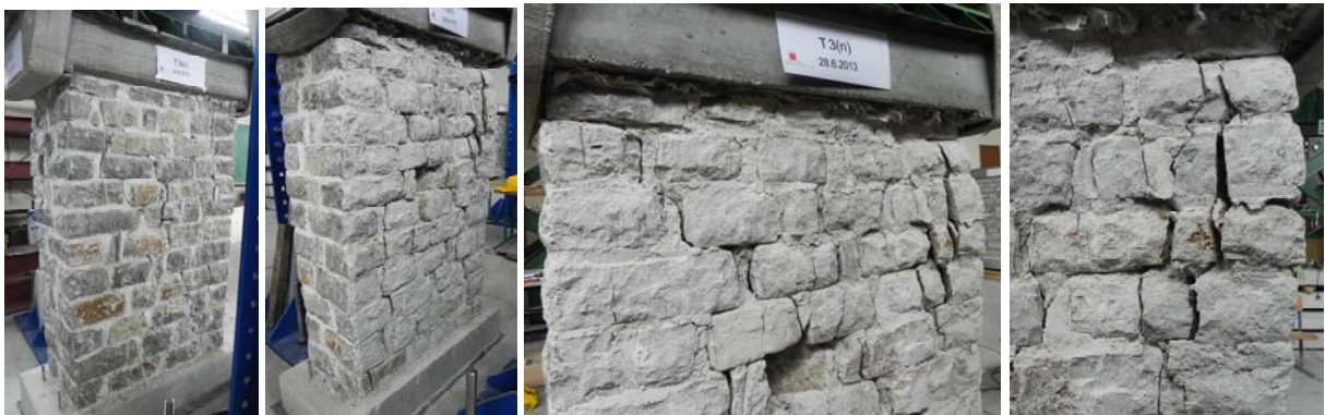
Figure 5.7: Damage of the wall obtained after test T3-n Slika 5.7: Poškodovanost zidu po testu T3-n
