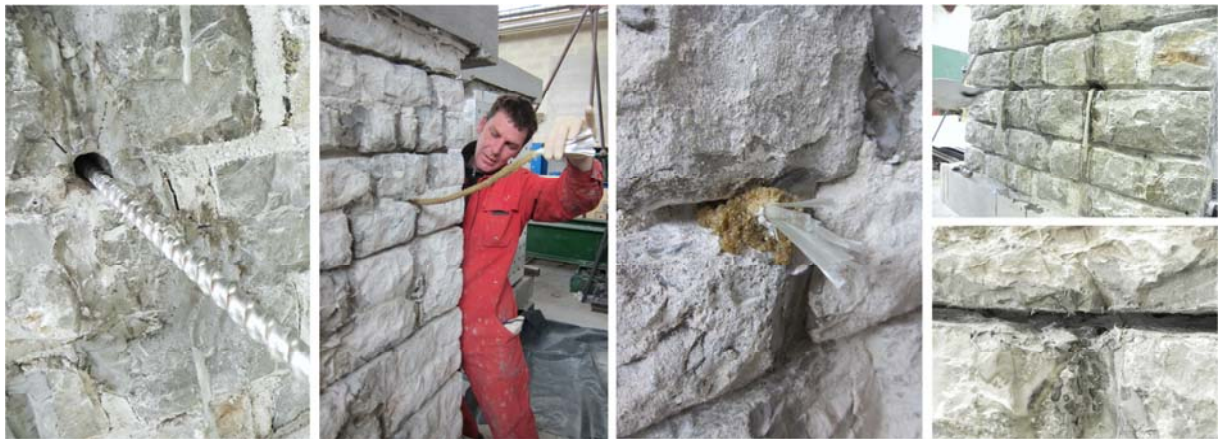
Figure 4.18: Drilling of the hole, the insertion of the impregnated cord coated in sand and sand "plug", transversal connection with impregnated cord (upper right) and with spread and fixed fibres (test 8 only, bottom right) Slika 4.18: Vrtanje luknje, povezovanje slojev zidu z impregnirano in s peskom posuto vrstico, pečeni "čep", prečna povezava z impregnirano vrstico (zgoraj desno) in razprostrta in prilepljena vlakna (samo test 8, spodaj desno)
