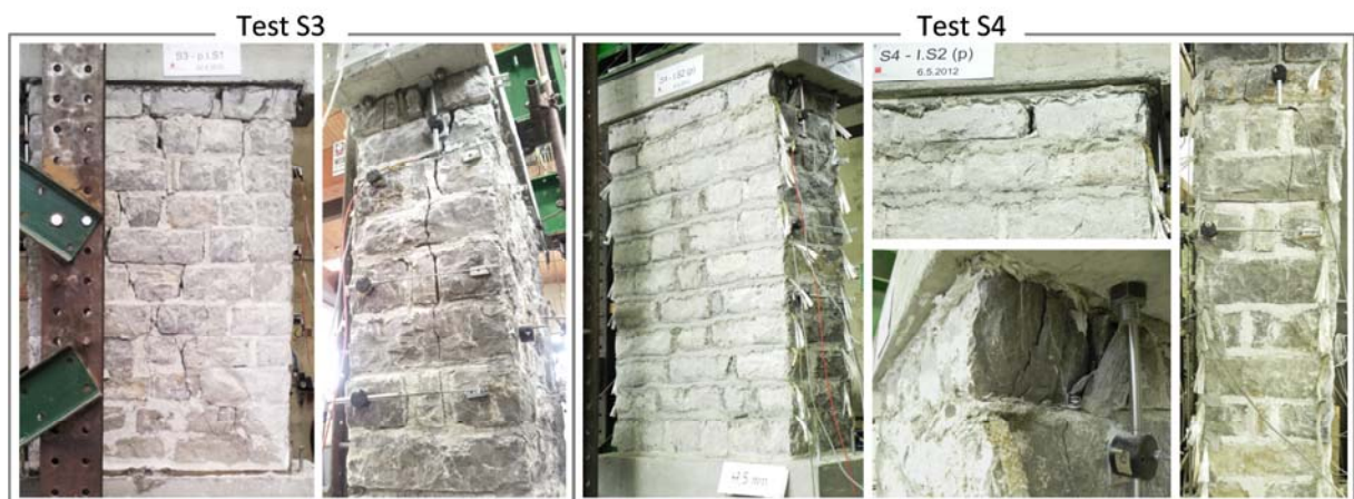
Figure 5.14: Rocking and minor shear damage on the wall after test S3 – I.S1(p) and rocking and toe crushing at test S4 - I.S2(p)
