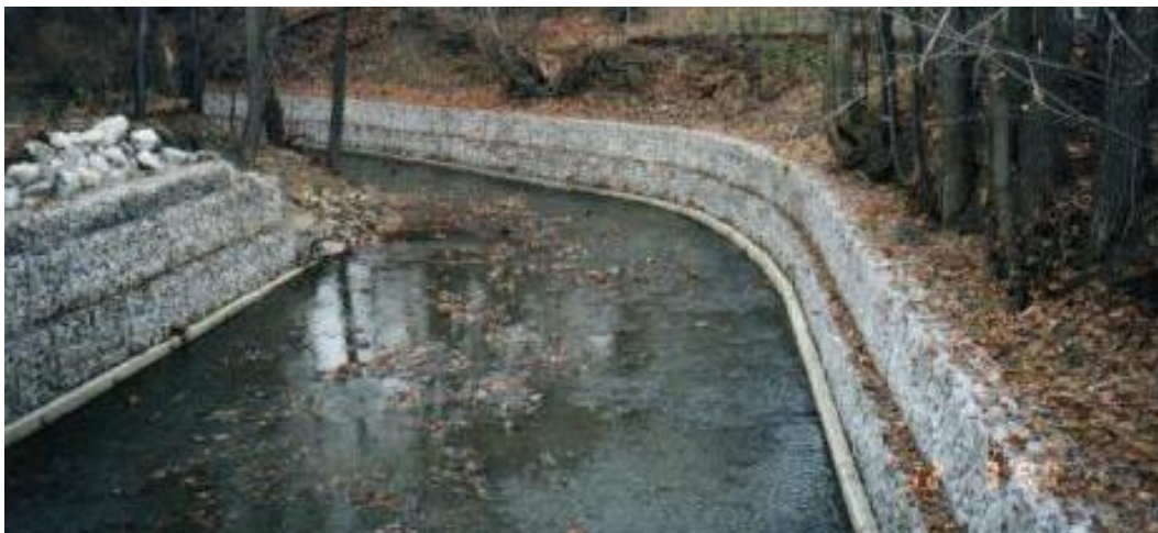
Slika 13: Brežine urejene z gabioni ( http://www.gabion1.com.au/gabion_erosion_control.htm )
