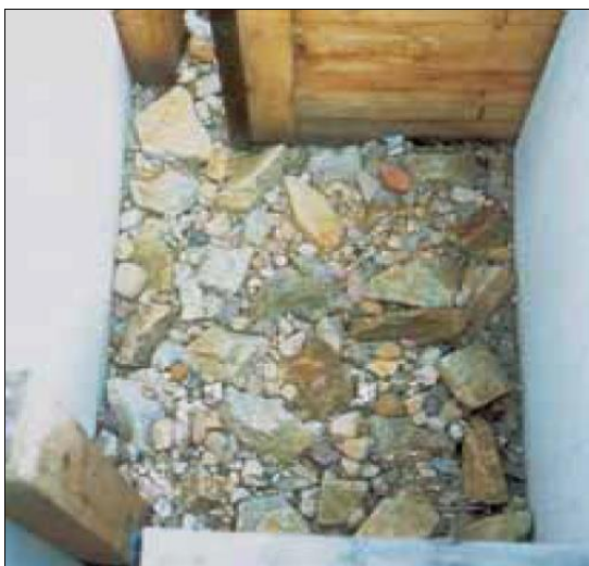
Slika 7: Grob substrat na dnu ribjega prehoda (Fish passes – Design, dimensions and monitoring, 2002)
