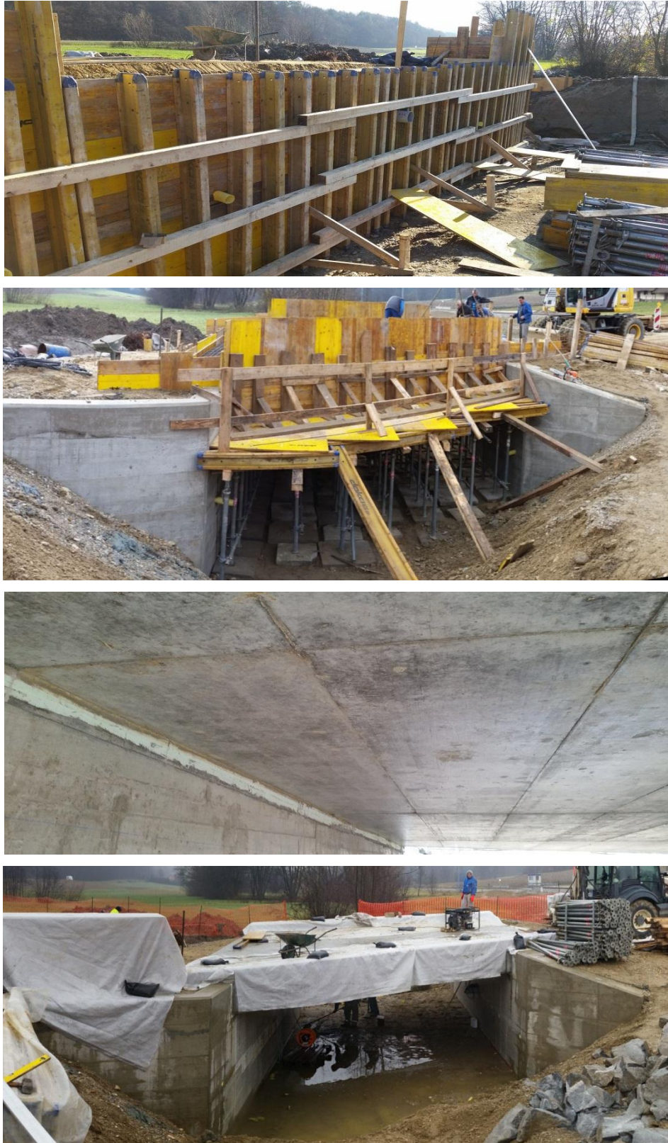
Slika 45: Izvedba opaževanja in betonskih del Figure 45: Formwork construction and concrete works
