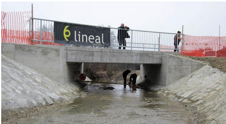
Slika 48: Struga vodotoka – kamen v betonu Figure 48: Stream culvert – rip rap structure
