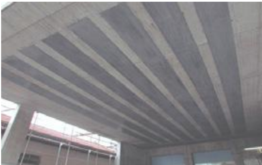
Slika 8: Karbonske lamele (Sika Services AG, 2014: str. 4)
