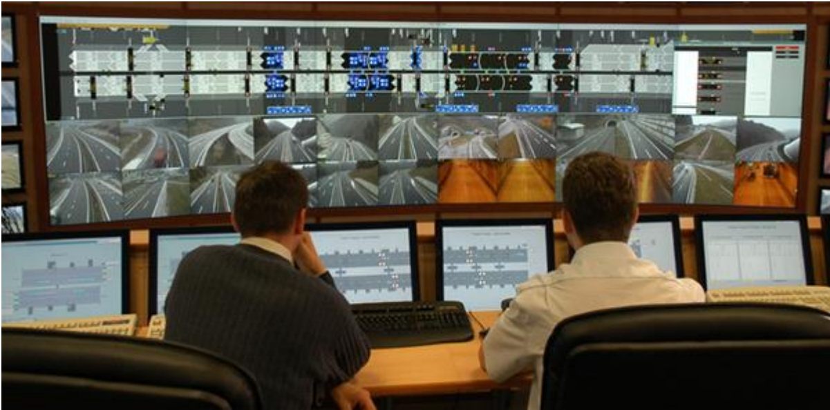
Slika 2-2: Nadzorni center za upravljanje sistema za nadzor in vodenje prometa Figure 2-2: Traffic Control Center as a part of the Traffic Management System
