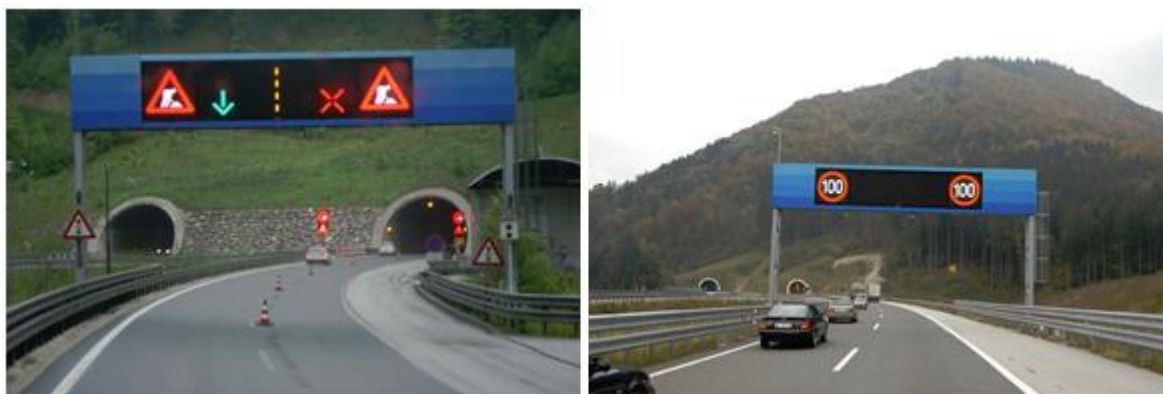
Slika 6-33: Dela na voznem pasu Figure 6-33: Road works on right lane
