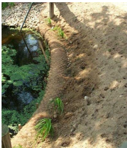
Slika 13: Zvitke iz geotekstila (Vir: http://www.co.winnepago.wi.us/lwcd/project/category/lwcd-project-category/shoreline-habitat-restoration )
