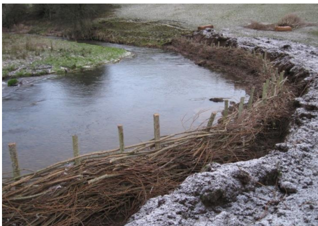
Slika 36: Gradnja živega plota (Vir: http://huttsatwork.files.wordpress.com/2013/02/willow-in-place-c-duncan-hutt.jpg )
