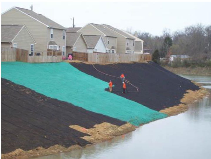
Slika 38: Prikaz vodne setve z dodatkom rastne pulpe (Vir: http://stopsilt.com/newimages/hydroseeding/RiverGlennGreenArmorSystem.JPG )
