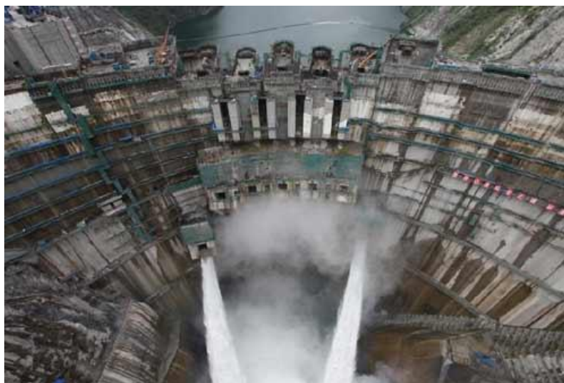
Slika 3: Najvišja ločna pregrada Jinping-1 305 m, Kitajska (Vir: http://journal.probeinternational.org/2014/02/03/jinping-i-dam-impoundment-linked-to-earthquakes/ )
