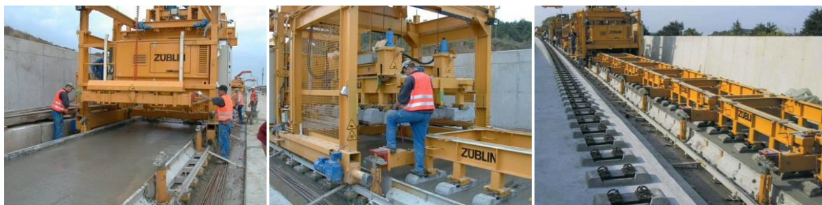
Slika 20: Postopek gradnje sistema Züblin (Vir: http://ict.uiuc.edu/railroad/CEE/pdf/PPT's/Spring09/Steidl%202-27-09.pdf (15.8.2013))
