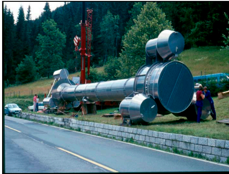
Figure 26: Aerator in Feldsee before put into place (Sampl, 2005)
