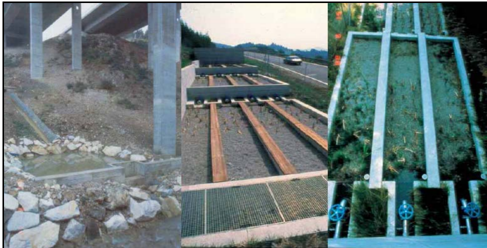
Figure 17: Constructed wetland along A2 motorway – Wörthersee region (Sampl, 2005)
