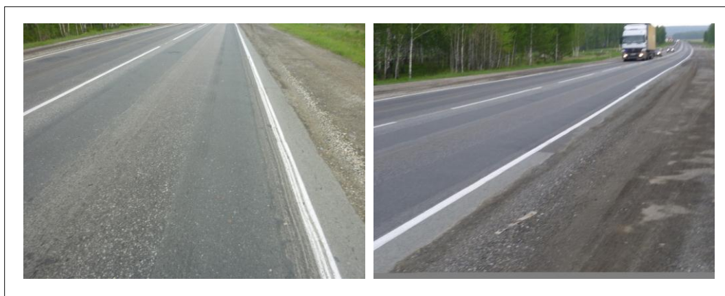
Slika 45: Sanirane kolesnice na cesti Federal Highway M5, Junij 2011 – Chelyabinsk, Russia (Cantat Associates Inc., 2012) [22]
