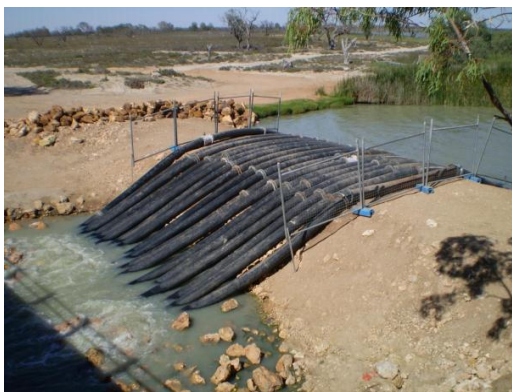
Slika 53: Prikaz navadnega sifona in shema obrnjenega sifona (vir: Dr. Stephen W. Hughes: A practical example of siphon at work, USBR – Design of small canal structures 1978)
