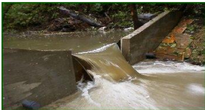
Slika 11: Ostrorobi preliv (U.S. Geological Survey, 2012)
