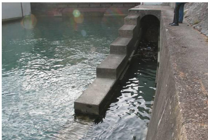
Slika 17: HE Dravograd – vhod v ribji prehod. Figure 17: HE Dravograd – fishway entrance.
