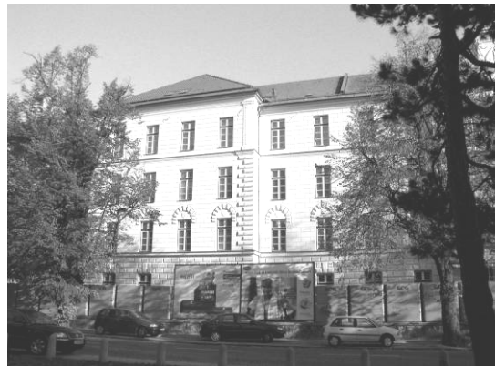
Fig. 1. North-east external view of the retrofitted museum building
