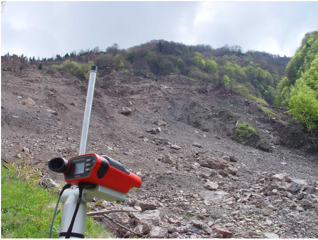
Fig. 1. Upslope view of the Strug rock fall source area from the fixed geodetic point “ST_KOS1” towards the scar of the rock fall.
