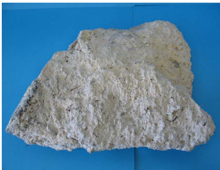
Figure 5-15. Deteriorated shotcrete with micro cracks.
