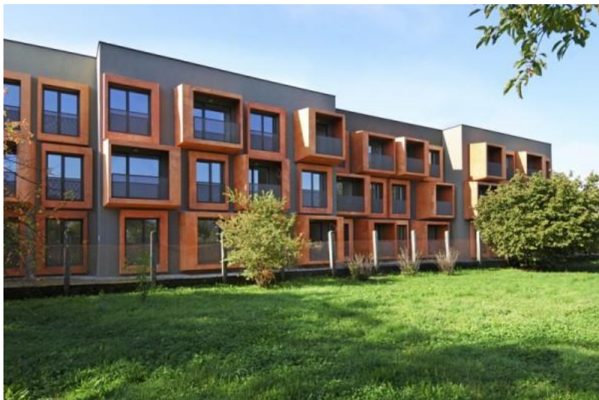
Slika 15: Stanovanjski objekt na Rudniku (Vir: http://timberland-boot-company.com/2011/10/page/4/ )
