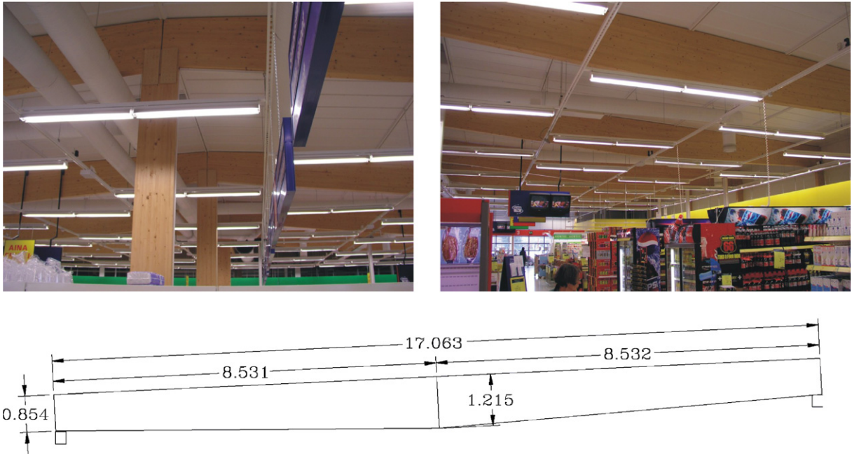
Fig. 1. Kokemäki K-Market and the geometry of the tapered glulam beam analysed in this case study.
