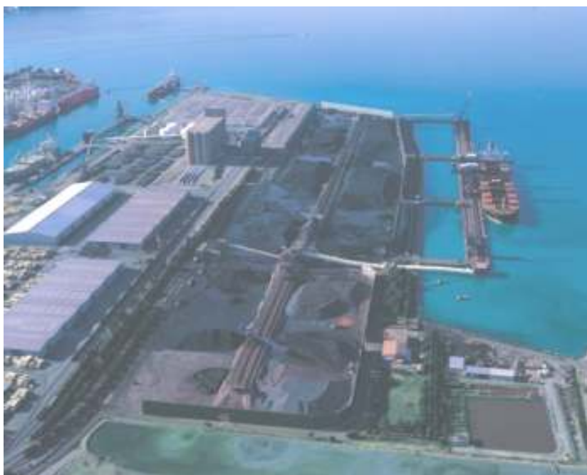
Slika 8: Evropski energetske terminal (Ponting & Pipenbaher Consultnig Engineers, 2007)
