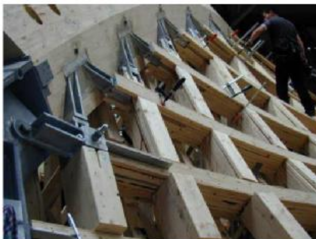
Slika 38: Rob lupine ob nosilcih in jeklene povezave med rebri ( http://timber.ce.wsu.edu/Resources/papers/3-6-1.pdf , pridobljeno 25.1.2011).
