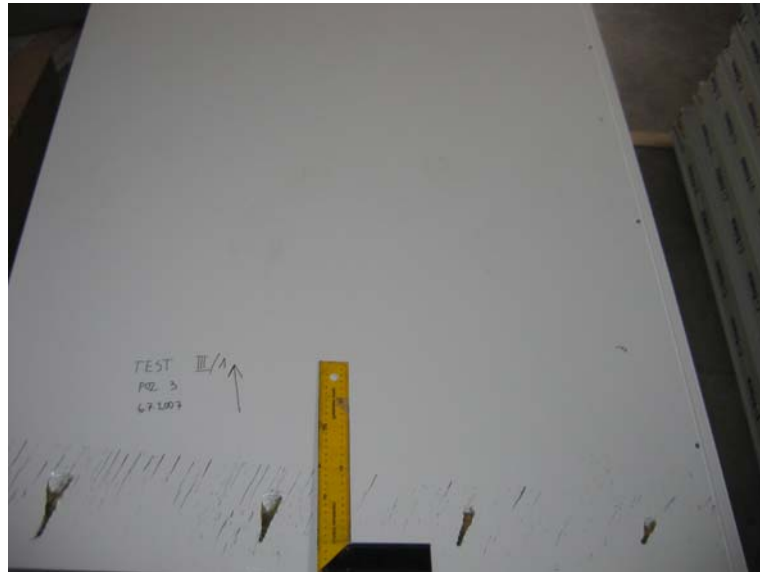
Slika B.12: Pretrg notranje pločevine zunanjega panela Figure B.12: The tear of the inner steel sheeting of the outer sandwich panel
