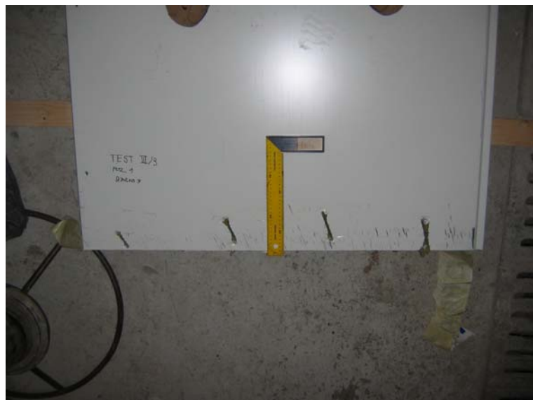
Slika B.19: Pretrg notranje pločevine zunanjega panela Figure B.19: The tear of the inner steel sheeting of the outer sandwich panel
